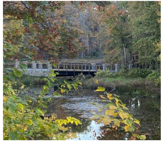
The new bridge behind The Rocky River Nature Center
